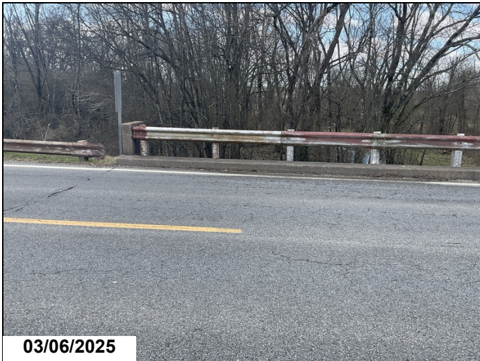
Rail has been repaired Span 1, left
