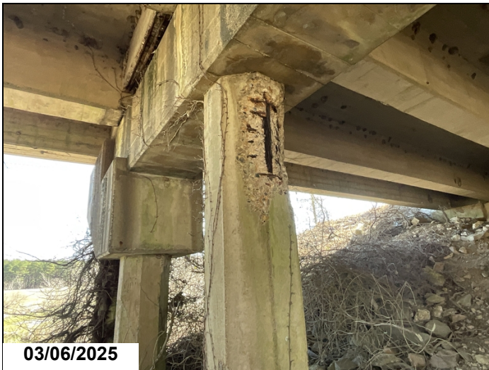
Bent 2, Pile 3, has 2' of spall with exposed steel with section loss to steel.
